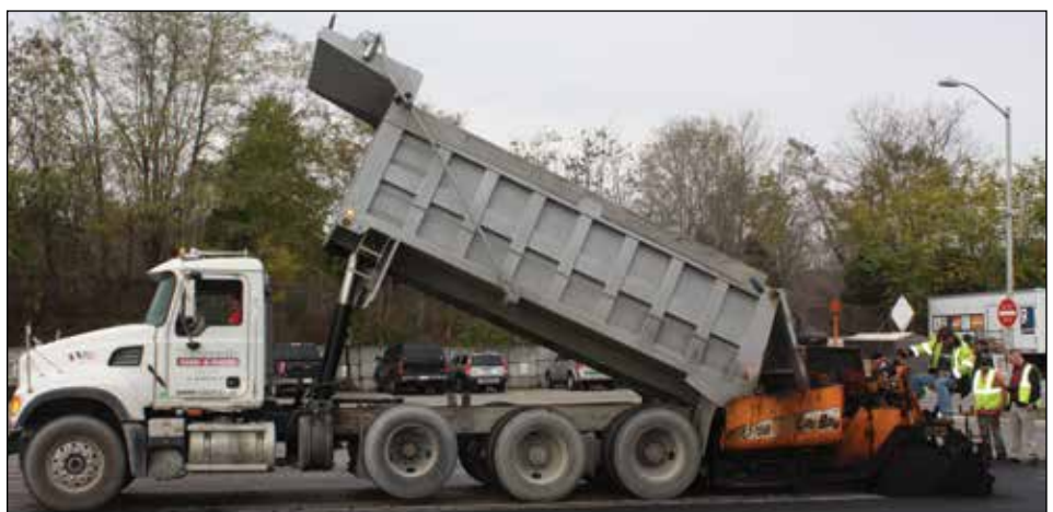
Benevento Companies' Mack truck feeds sustainable asphalt mix to U.S. Pavement Services' LeeBoy 8510B Paver at the recycling center. By Paul Fournier
