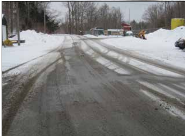
This photo shows a street plowed with the multi-sectional carbide blade on the left and a traditional steel blade on the right.
