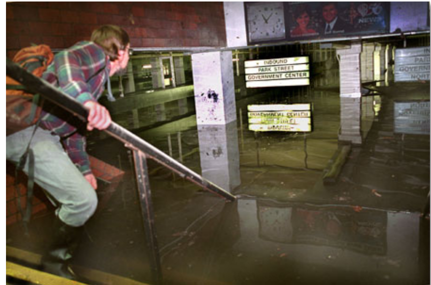
Flooding at Kenmore Station (Green Line)
