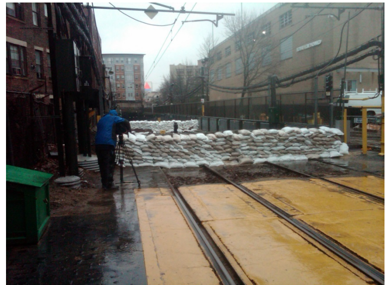
Sandbag barrier at Fenway Portal (Green Line) during heavy precipitation event, March 2010
