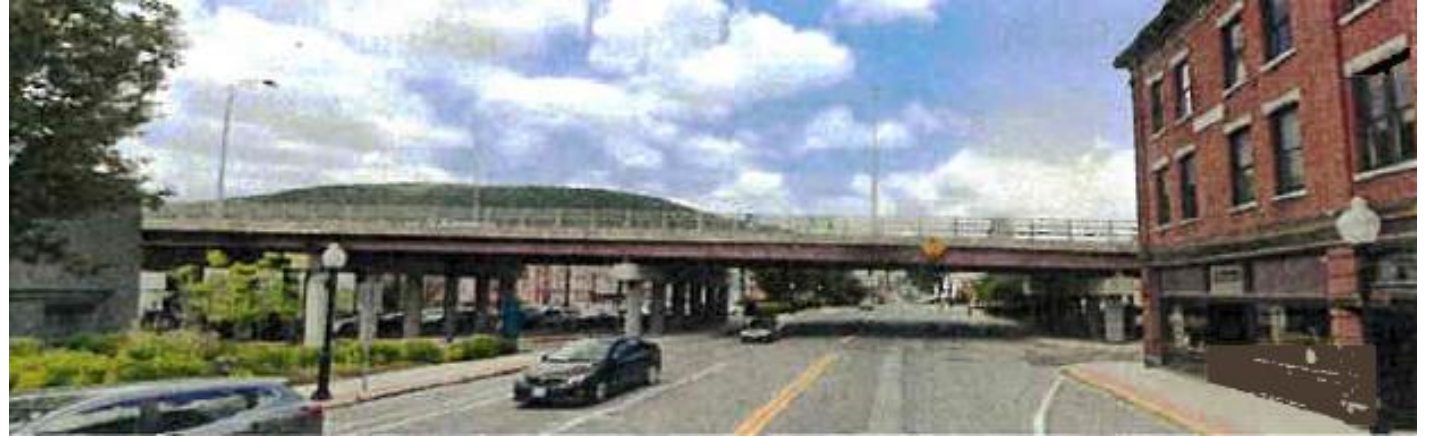
Source: City of North Adams, Route 2 Overpass RCP Application
