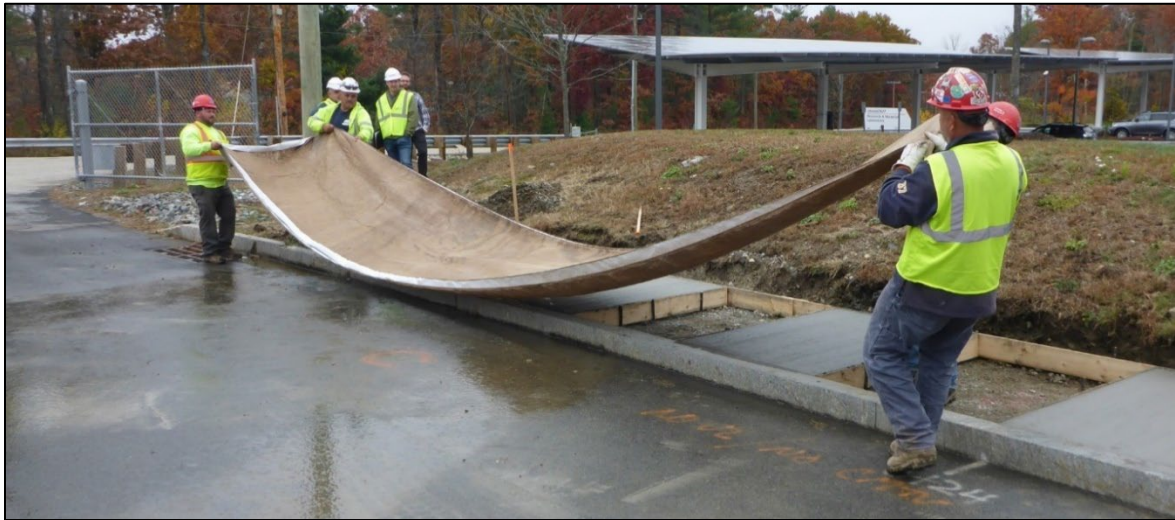
Figure 5.8: Application of saturated cover
