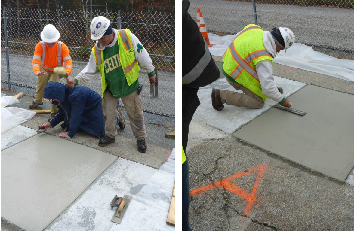
Figure 5.5: Prohibited practices panels—blessing (left) and steel trowel (right)
