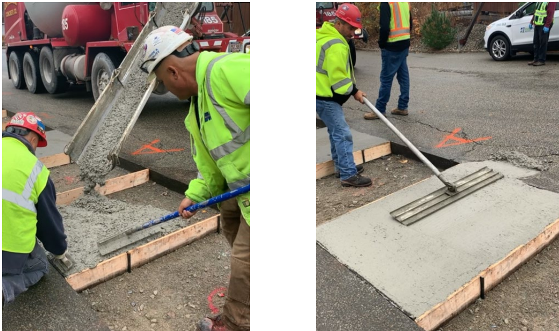
Figure 5.3: Concrete placement into form (R); bull floating using magnesium float
