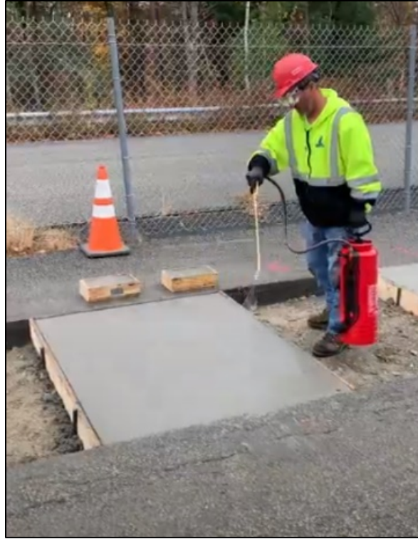
Figure 5.10: Water sheen observed on panel as curing compound is applied
