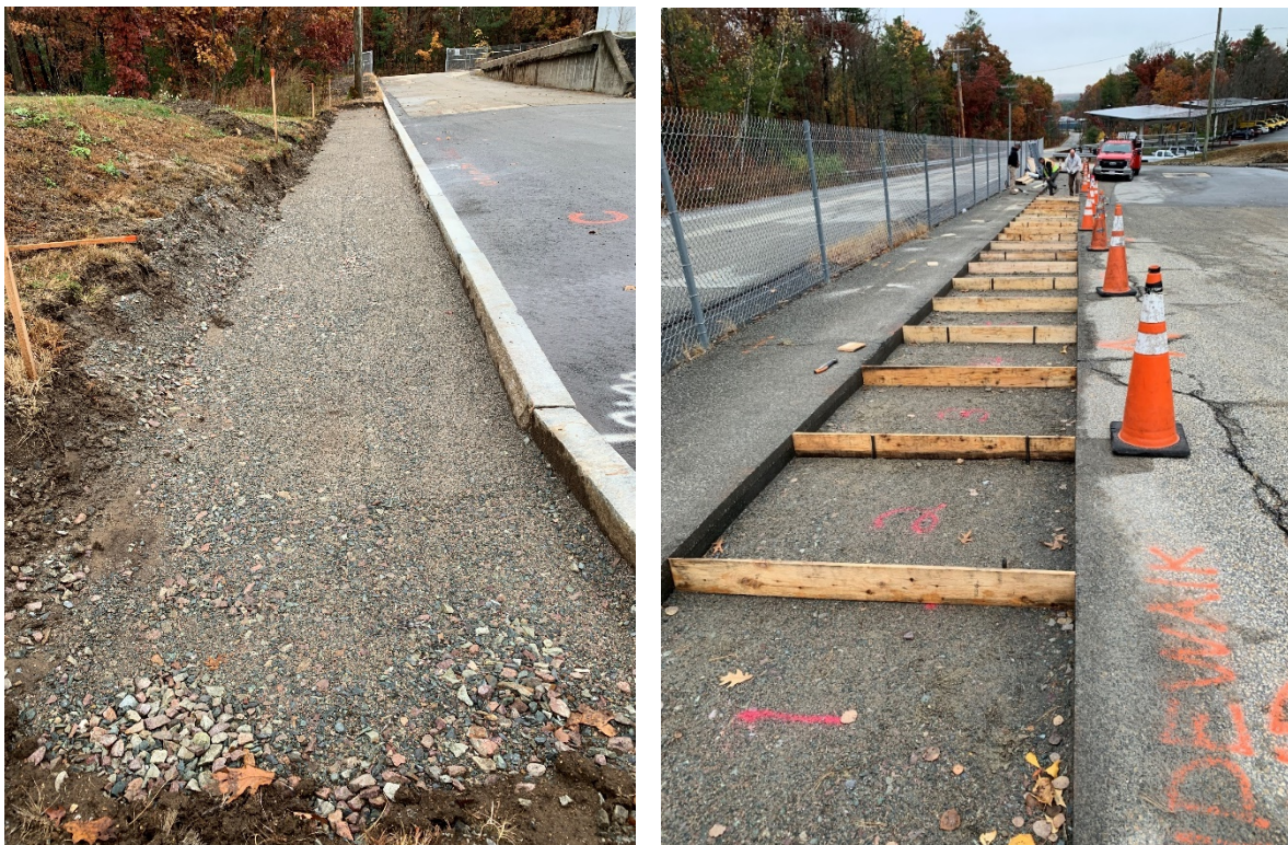
Figure 5.2: Compacted subgrade in Panel Groups C, F, I (left); Panel Groups A, D, G, B, E, H (right)
