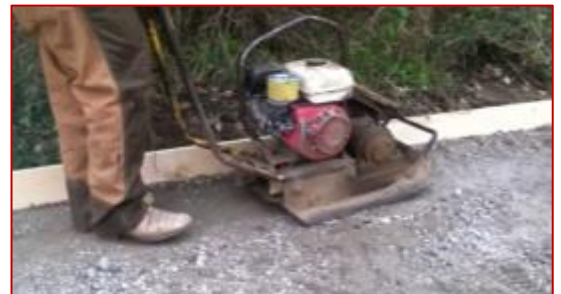
Compaction is critical for a good base
