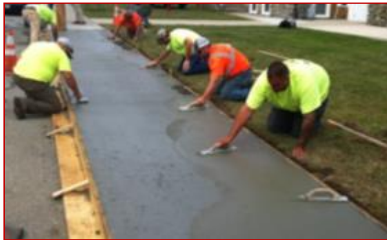
Cutting the edge and floating the surface
