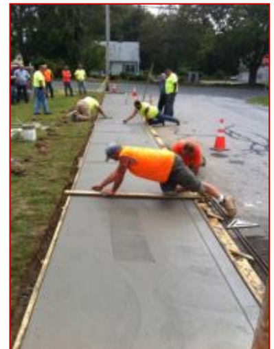
Cutting the center joint
