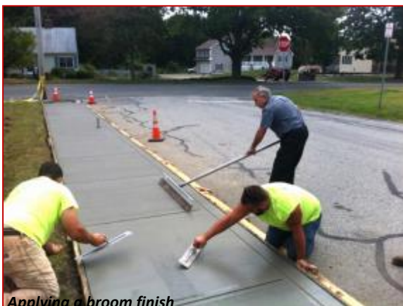
Applying a broom finish
