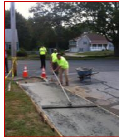
Bull floating the concrete
