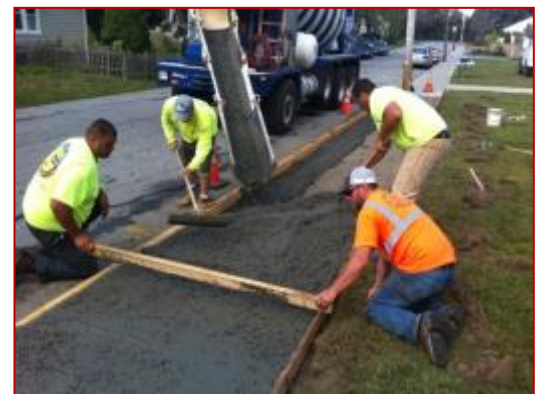
Pouring and leveling the concrete
