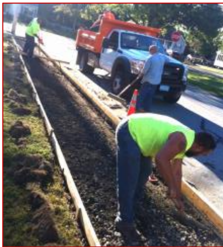
Preparing the base
