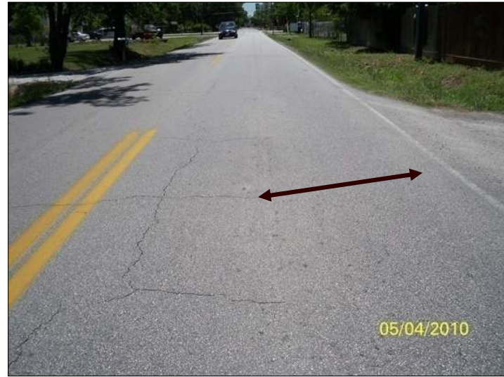
Van Hut Road 4 years after install.
