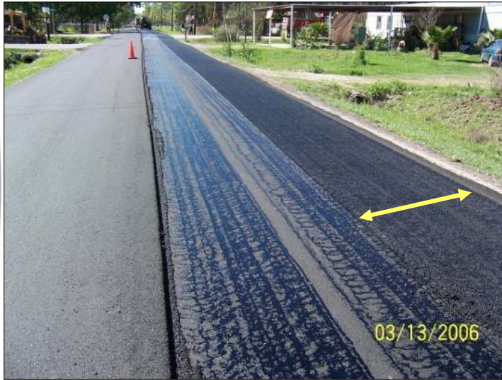
Van Hut Road GlasGrid® placed on shoulder.
