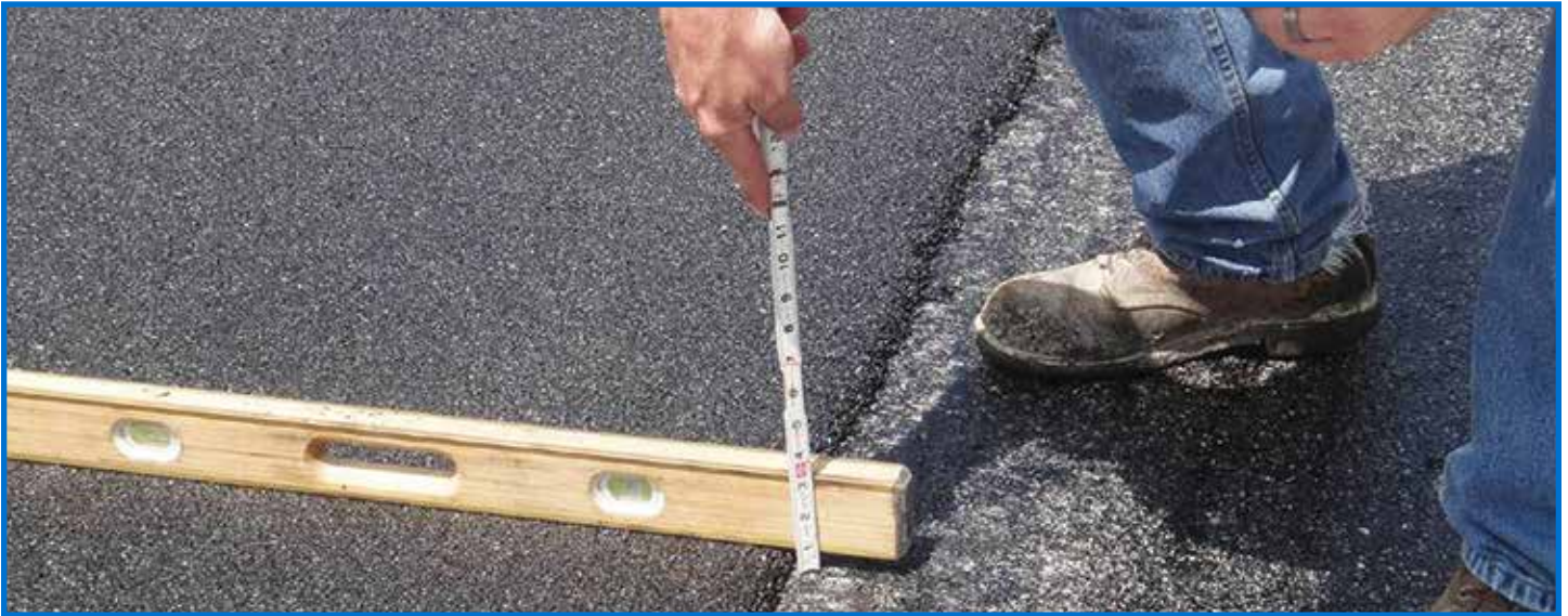
Thin HMA overlays are an important pavement preservation tool, with their design optimized for 3/4 to 1 1/2 inches in depth Photo courtesy of Texas Transportation Institute
